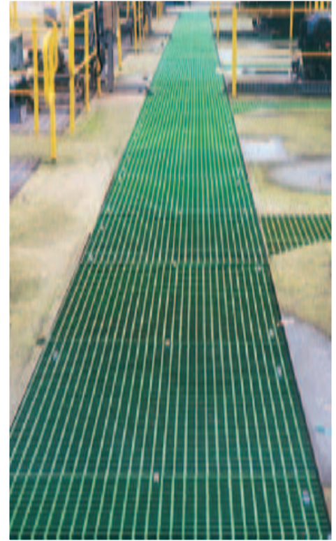
Fibreglass Grating replaces corroded steel mesh covers
