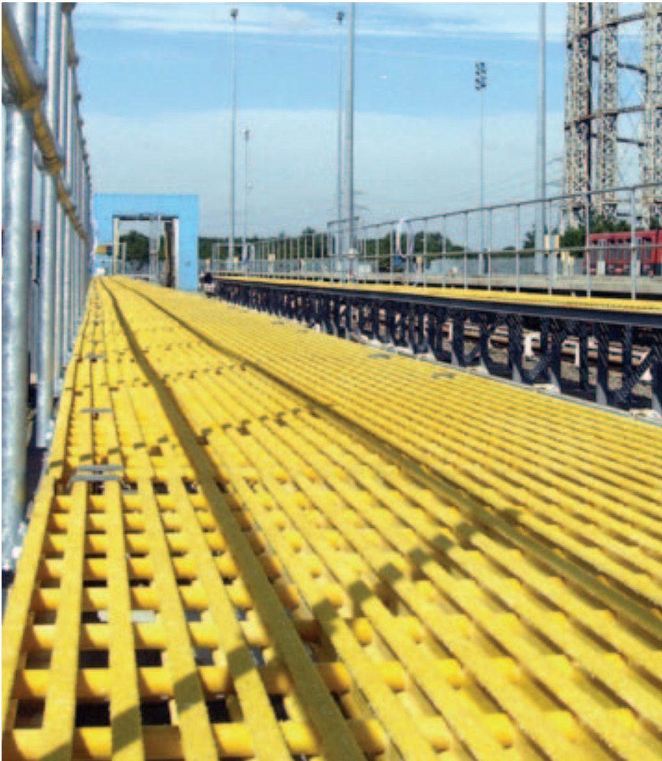
Grating replaces steel construction wash bay walkway for Docklands Light Railway
