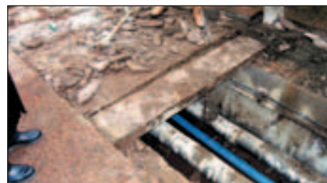
Removal of concrete covers prior to installations
