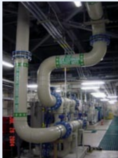
Process cooling water with [β]-PP-H (Polypropylene) in Power Industry .
