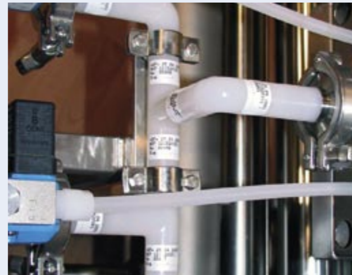
SYGEF® PVDF with BCF® welding in Pharmaceutical .
