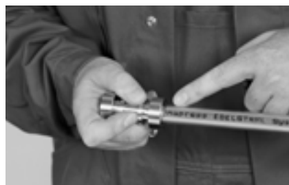
Figure 10.0-13 Pushing mapress pipe into pressfitting
