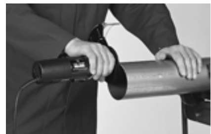
Figure 10.0-8 External deburring with RE1 electric pipe deburrer
