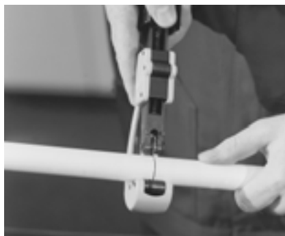
Figure 8.0-26 Cutting to length with pipe cutter
