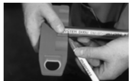
Figure 10.0-9 Marking insertion distance
