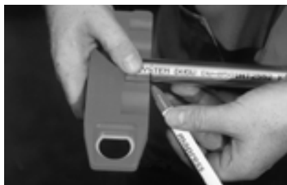
Figure 8.0-7 Marking insertion distance
