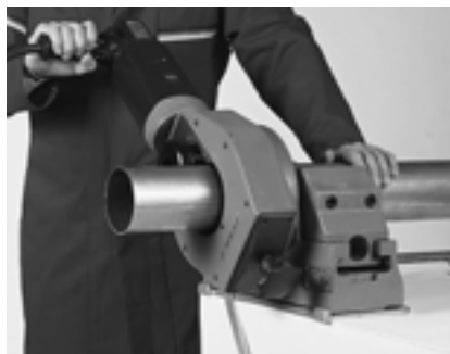
Figure 8.0-4 Cutting to length with electric saw
