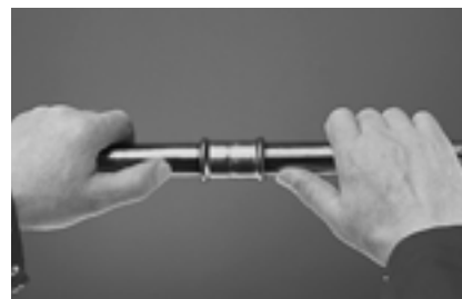
Figure 8.0-12 Pushing mapress pipe into pressfitting
