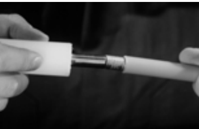
Figure 8.0-22 Introducing reinforcing sleeve
