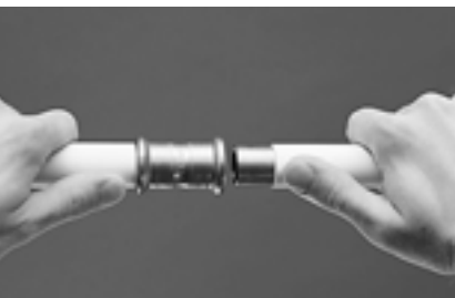
Figure 8.0-33 Pushing CARBON STEEL pipe into pressfitting
