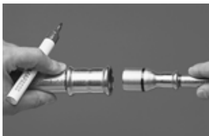
Figure 8.0-9 Pressfitting with plain end and insertion distance 'i' mark
