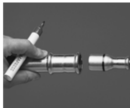
Figure 8.0-38 Pressfitting with plain end and insertion distance 'i' mark
