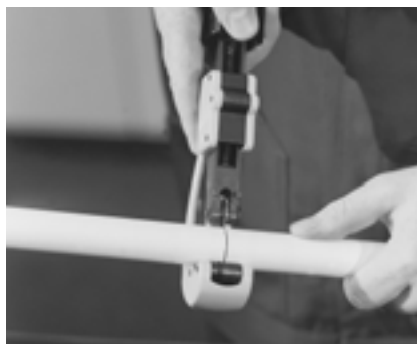
Figure 8.0-41 Cutting to length with pipe cutter
