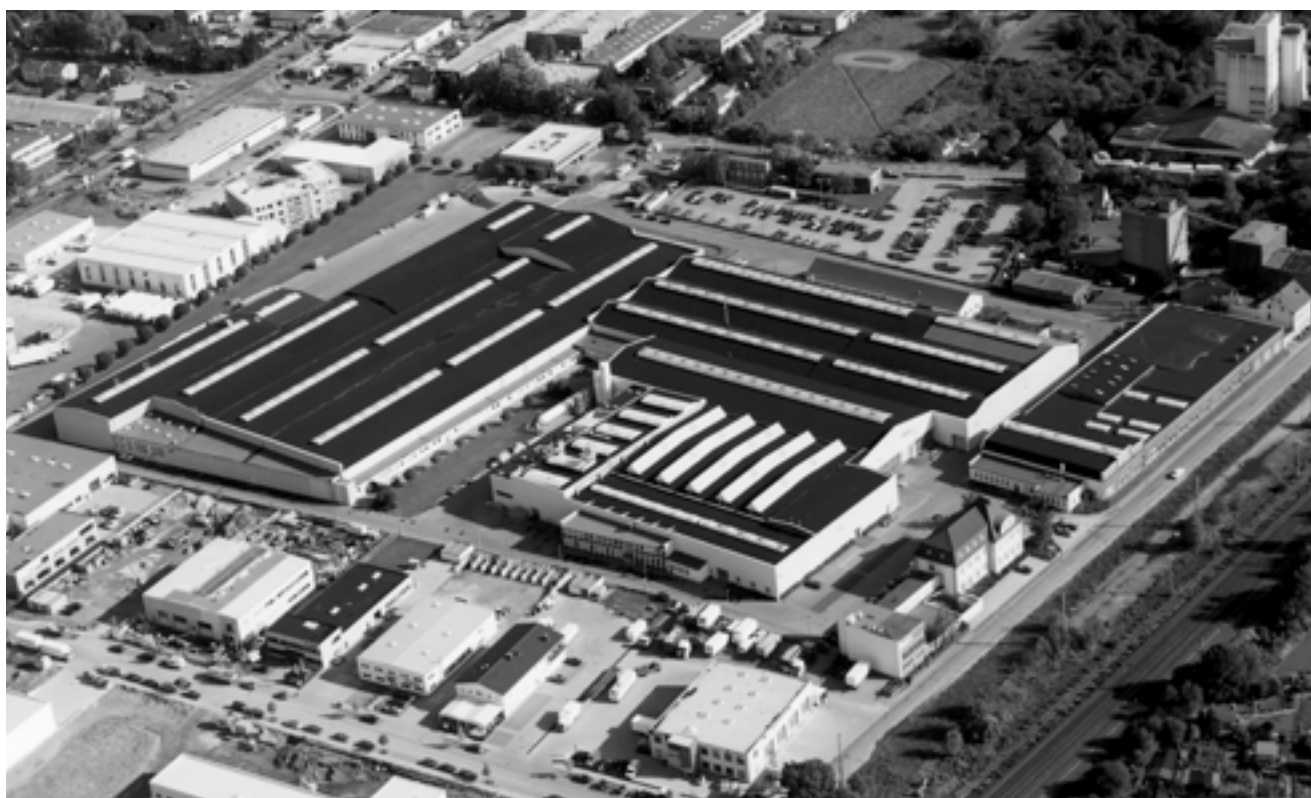
Figure 1.0-1 Aerial photograph of Geberit Mapress GmbH facilities
