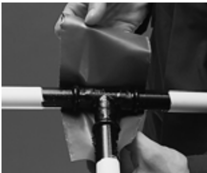
Figure 9.0-2 Anticorrosion taping of connection
