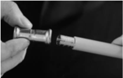
Figure 8.0-24 Pushing EDELFLEX pipe into pressfitting
