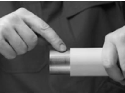
Figure 8.0-32 Marking insertion distance 'i'
