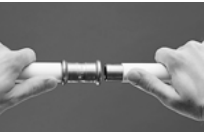
Figure 8.0-49 Pushing DIN EN/DVGW copper pipe into pressfitting
