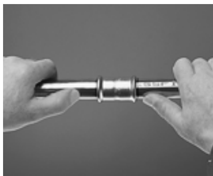
Figure 8.0-40 Pushing copper pipe and pressfitting together
