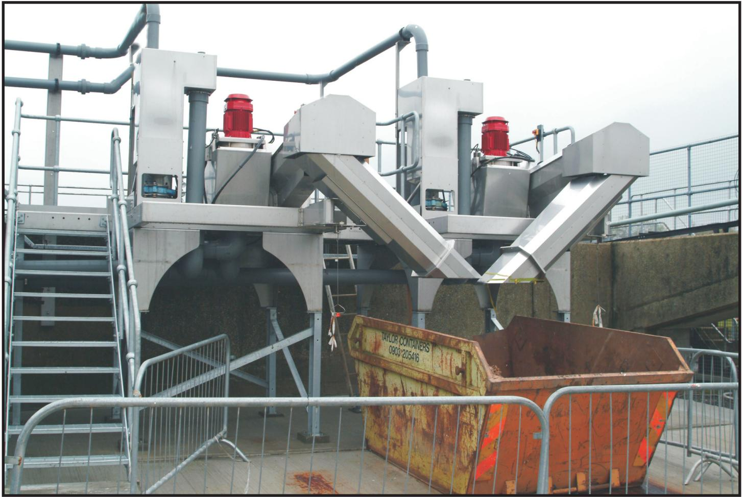
The installation serves a population of over 70,000 and consists of a 2000 Lisep Package with 402 Macipump, LS403 Liquid Separator, 403 Lipactor & Slave Grit Macipump 300.
