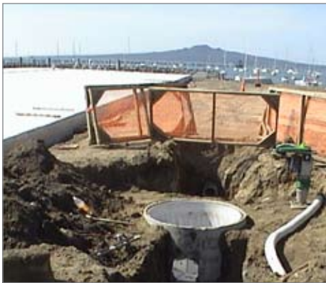
The low headloss of the Up-Flo Filter suited the Marina's shallow drainage system.
