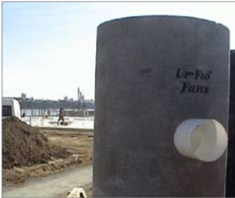
The Up-Flo Filters were delivered to the site in standard 4-ft diameter manholes to make it easy to readily install the devices into the drainage network.
