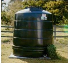
This requirement does not apply when a well, pond or stream is used as the water source, but if the capacity of the well is small then it may be necessary to pump it throughout the day into a tank to feed the night operating watering system. Where a storage tank is necessary, its capacity will depend upon the relationship between the overall demand of the irrigation system, the capacity of the water supply and the peak design demand of the system.
