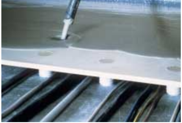
Hohlraumboden Typ Cavopex / Cavopex type cavity floor / Plancher cellulaire de type Cavopex
