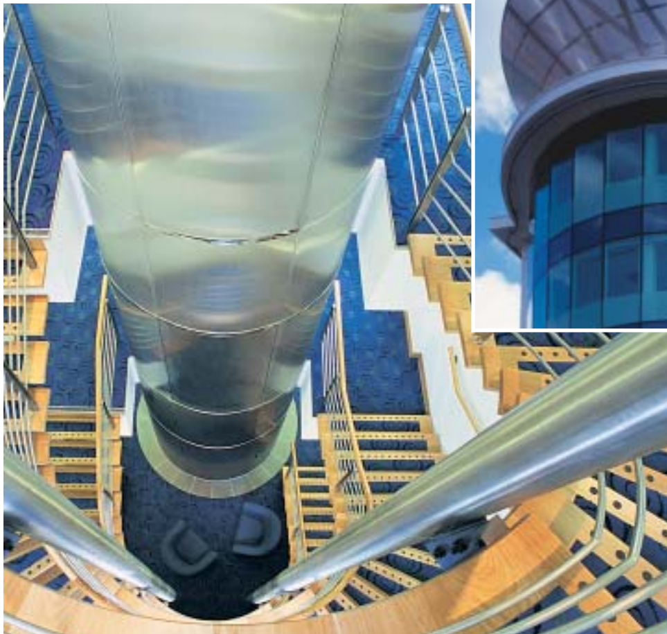
Stainless steel lift shaft cladding.
