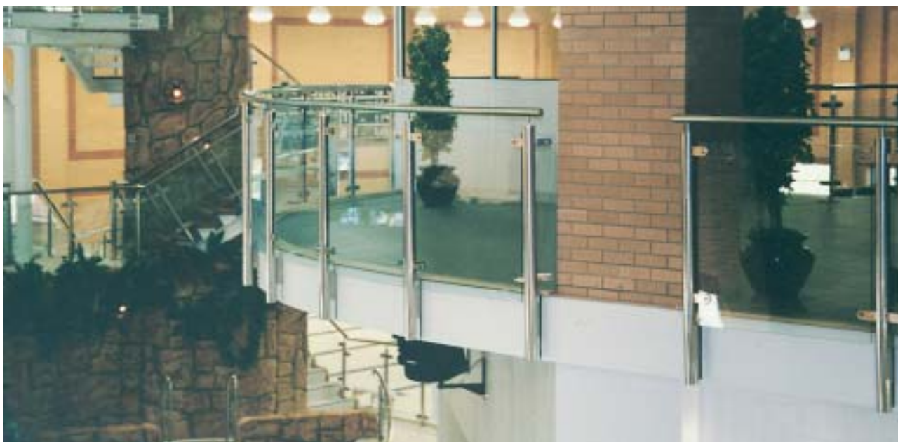
One of our projects. Curved stainless steel balustrading to viewing gallery complete with toughened glass infill panels.
