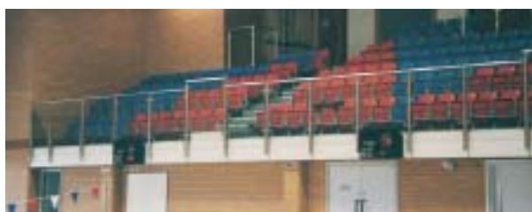
Swimming Pool spectator balustrading manufactured from 316 grade stainless steel complete with toughened glass infill panels.
