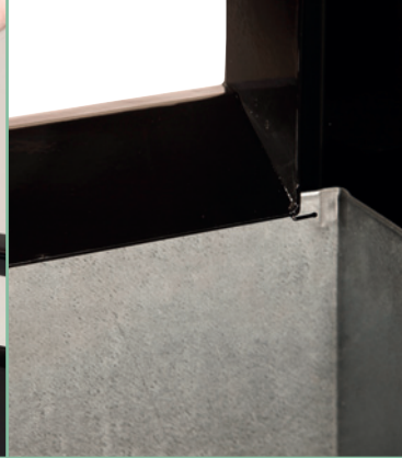
Deep aperture opening overhanging liner.
