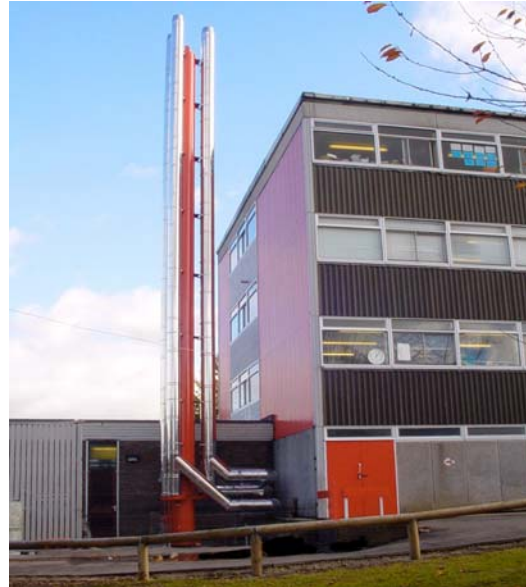
16m high mast with HT twin wall flues Smithwood School - Solihull
