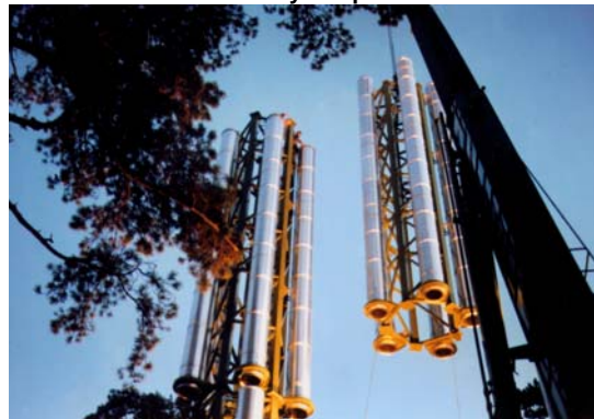
50m high mast BBC Head Quarters, South Wales
