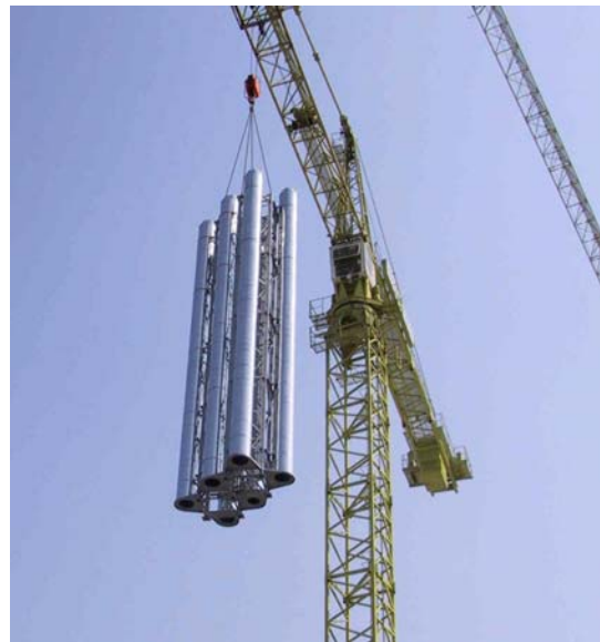
33m open lattice mast Bromley Hospital
