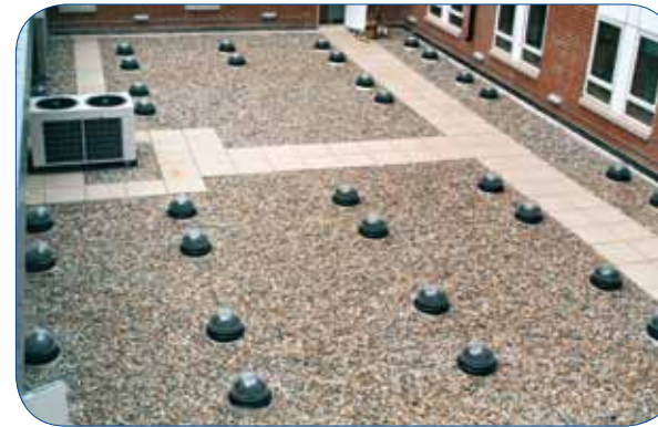
Centre right & lower right: Lewisham Police Station, London, where 50 No. 330mm diameter Sunpipes were installed to the cells of this high security building. The Sunpipe systems were fitted with vandal resistant top domes and security bars. Stainless steel ceiling trims were fitted with security screws.
