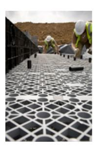
Working closely with the groundwork contractor, W Longs, Polypipe WMS supplied 3000 cells to provide an attenuation solution to manage surface water run-off from both hard standing and roof areas. Installation guidance was also provided to W Longs' on-site team. Following consultation with both the MoD and W Longs, Polypipe WMS also designed a manifold system to improve hydraulic performance of the overall attenuation solution.
