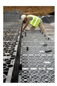
The original project specification included a concrete box culvert. However, following the main contractor's issues with rising material costs and concerns over the performance of the product in times of high-flow water run-off, Polypipe WMS was approached to design a solution capable of storing the required water capacity whilst accommodating difficult site constraints.
