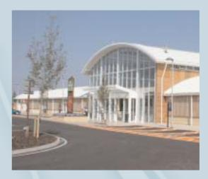
requirement Rigidal are able to offer both smooth and crimp curved options together with profiled closure pieces, flashings and mitred units.
