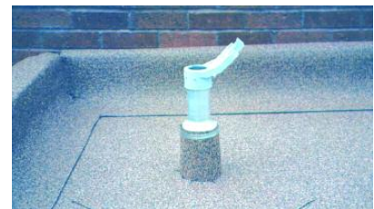
2. Waterproof the base and upstand.
