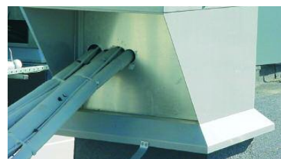
4. Cut pull-out panel to pipe work.
