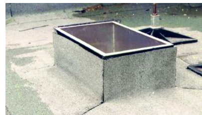
2. Waterproof the base and upstand.
