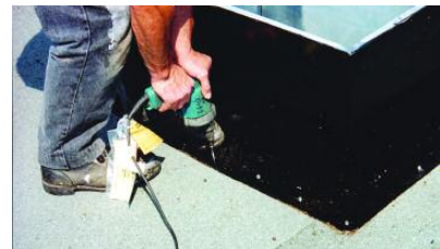
1. Mechanically fix the base unit to the deck.
