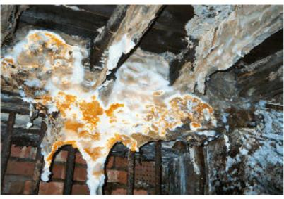
A further feature of the fungus is the formation of 'strands', thick walled structures which develop in the fungal growth. These are resistant to desiccation and carry nutrients from the food source to the growing tips of the fungus when the organism is growing through or over nutritionally inert materials, eg, masonry, soil. They support the spread of the growth. However, without a source of food growth is terminated.
