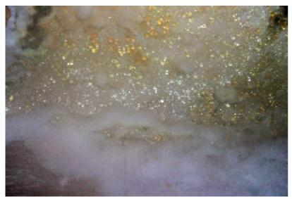
The first evidence of the existence of an outbreak of dry rot is often the sudden appearance of a fruiting body (sporophore), or the shrinking/distortion of timbers. This latter feature can be quite dramatic and sudden, the change from dimensional stability to instability of the wood visually taking place relatively suddenly; this explains the apparent sudden appearance of dry rot frequently reported. It should be noted, however, that fruiting bodies are not always formed.
