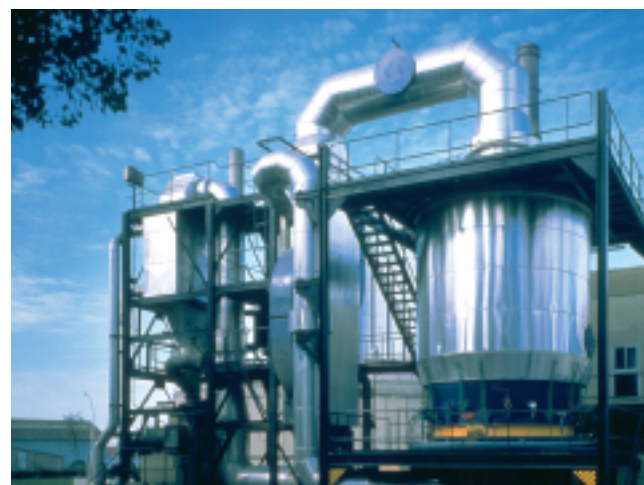
Le Havre (France) – The PYROFLUID® incinerator
