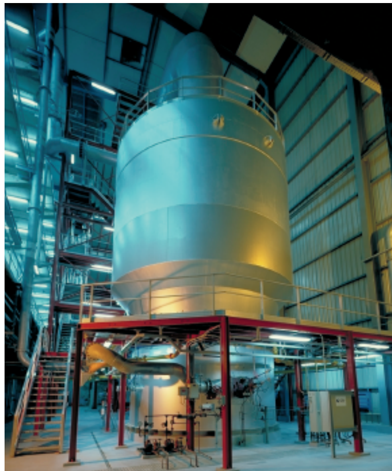
Saragossa (Spain) – The PYROFLUID® incinerator
